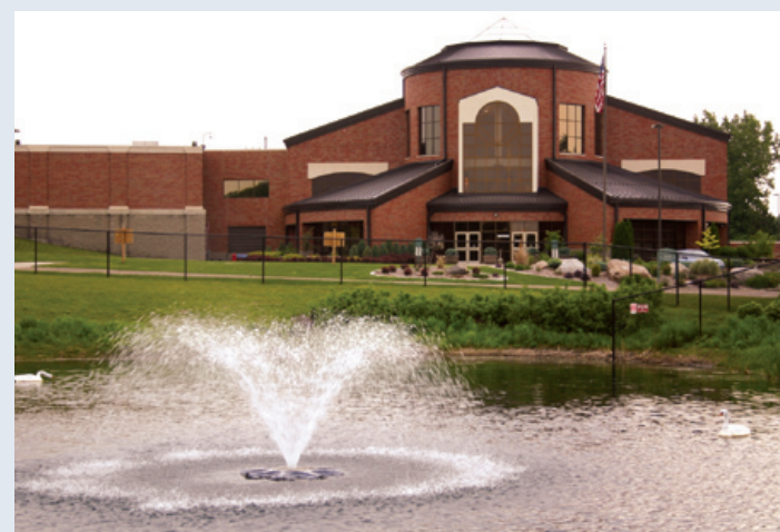
Eden Prairie Water Treatment Plant
