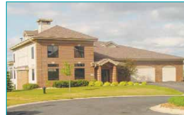
Several other cities have built house-like structures around wells. This water treatment plant is located in Savage.
