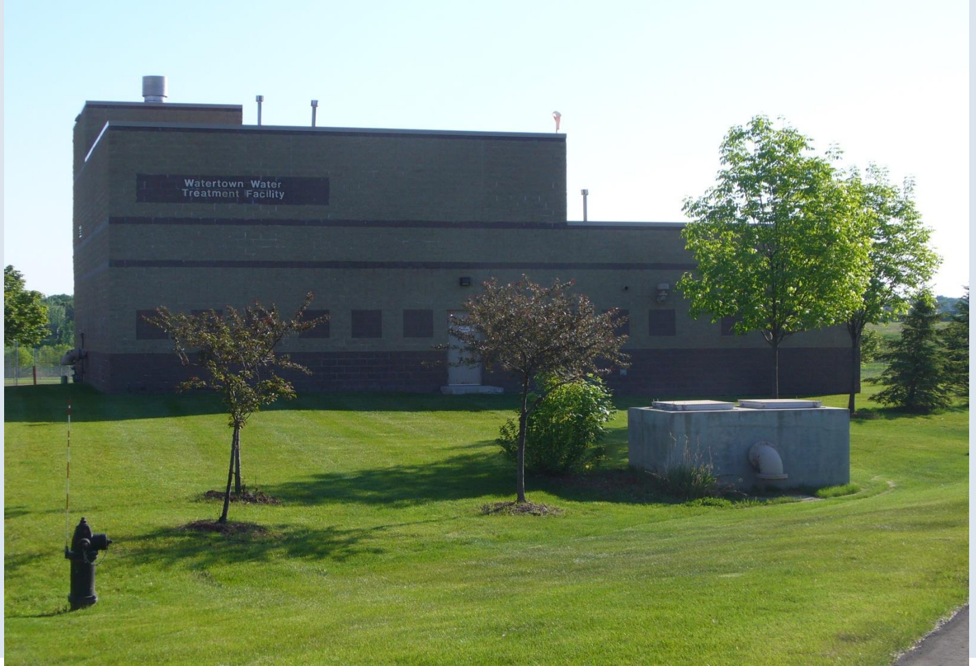
Watertown Water Treatment Facility
