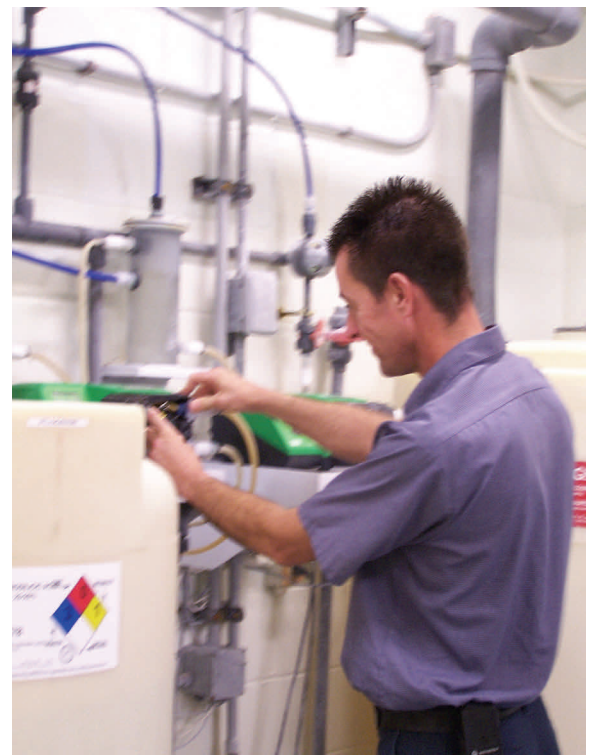
Utilities crew member Brian Vos works on the fluoridation equipment
