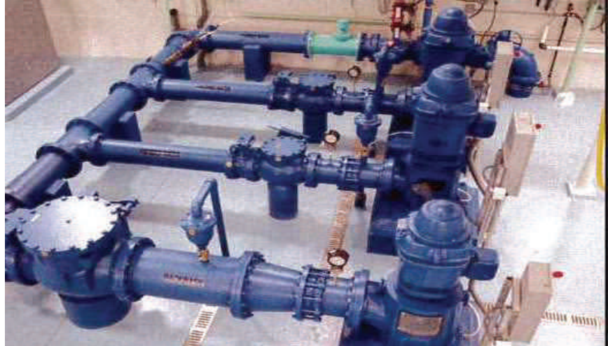
High Service Pumps
