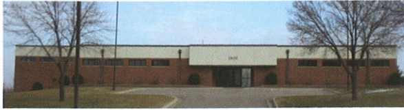
Maple Grove Water Treatment Plant
