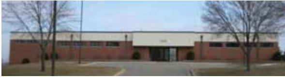
Maple Grove Water Treatment Plant
